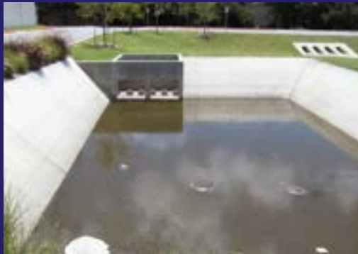
Example: Stormwater Ponds
